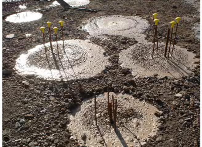
*Expanded Head VCC's with Reinforcement steel*
