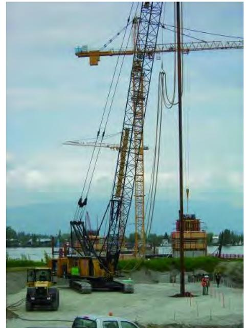
1. Using the rigs pull down force, water jetting and sustained vibration allows the probe to penetrate to the design depth.
