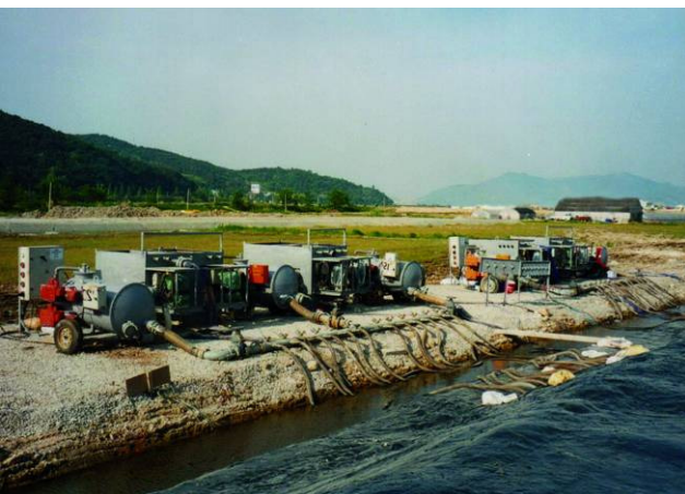
Menard Vacuum Consolidation Process
