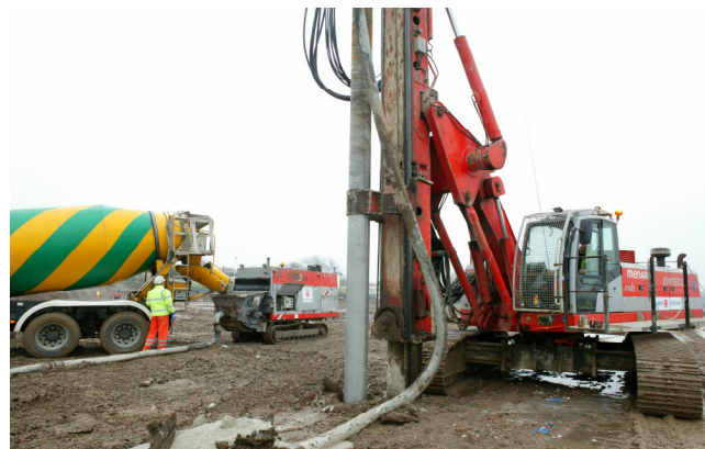
CMC's installed for building slabs or rail/road embankments
