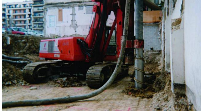
CMC's installed close to existing building foundations
