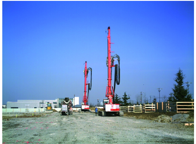
Stone Column and CMC rigs in operation building Bi-Modulus Columns
