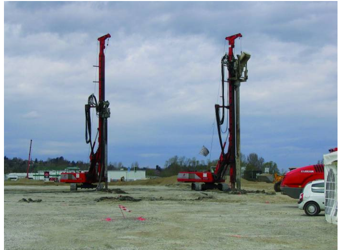
Stone Column and CMC rigs in operation building Bi-Modulus Columns
